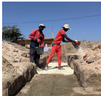
Step 1 Digging foundations
