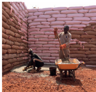
Step 4 Pouring cement for flooring
