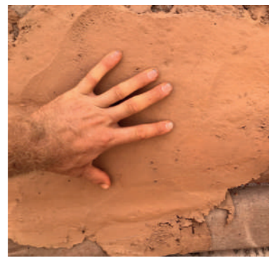
Step 4 Applying coating layer
