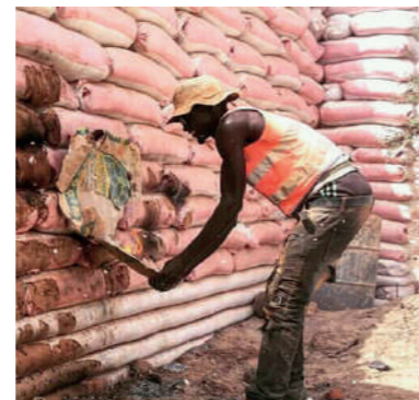
Step 3 Burning earth-bags to receive the coating layer
