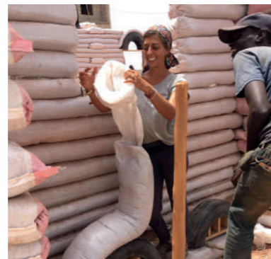
Step 2 Piling earth-bags to compose walls and furniture
